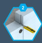
STRIPPING Cut off the excess insulation.
