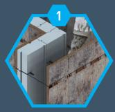
PANEL INSTALLATION Inside the traditional wood formworks. Before the concrete casting.
