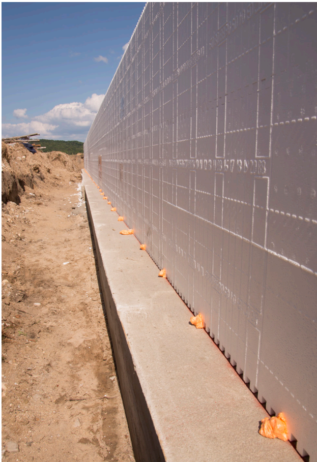
Figure 4.3.2 First two courses leveled and spot glued using foam adhesive. Use small amounts to prevent lifting the wall. Add additional adhesive after spot glue sets if desired.
