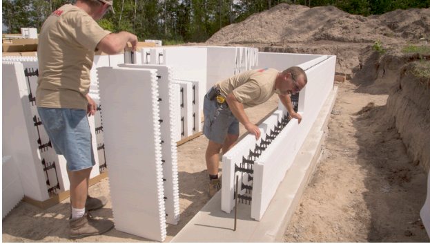
Figure 4.3.1 Stacking first two courses starting from a corner and working in a single direction.
