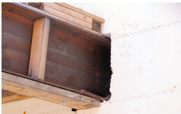
Figure 5.11.1 Steel beam placed in ICF beam pocket.
