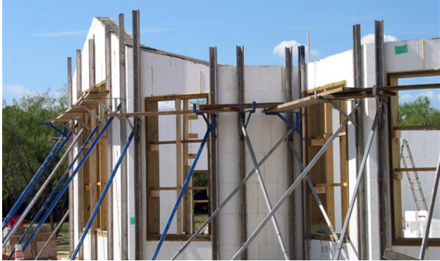
Figure 9.6.2 More Secure Outer Bracing
