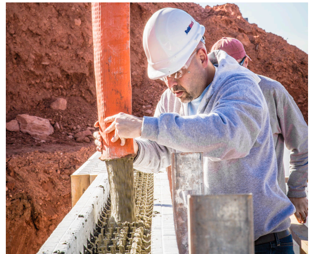
Figure 3.2.2 Pouring concrete into an ICF basement using a pump truck and flat hose.
