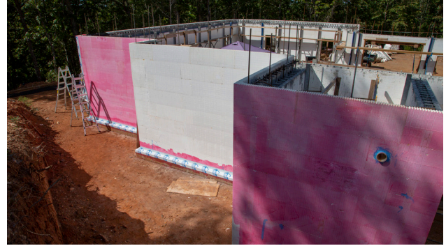
Figure 6.4.4 Detail strip attached along footing and corners. Walls partially primed for Home Stretch membrane installation. Membrane is attached to the ICF wall and sealed to the top of the footing.
