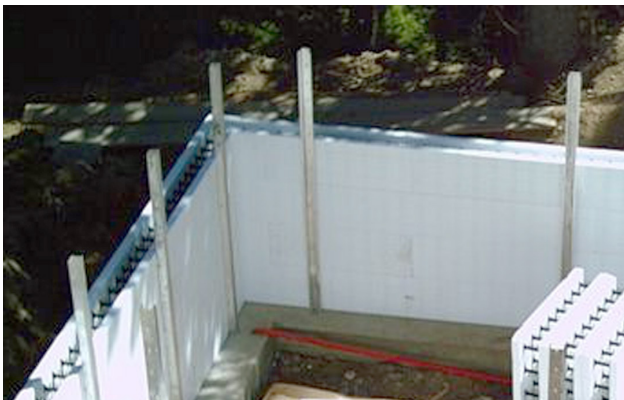
Figure 9.6.3 Minimal Inner Bracing
