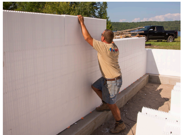
Figure 4.5.1 Stacking ICF walls using spot glued dry set method.
