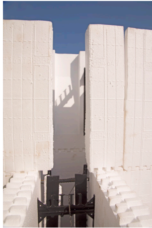
Figure 5.5.5 Intersecting wall opening alternating form placement.
