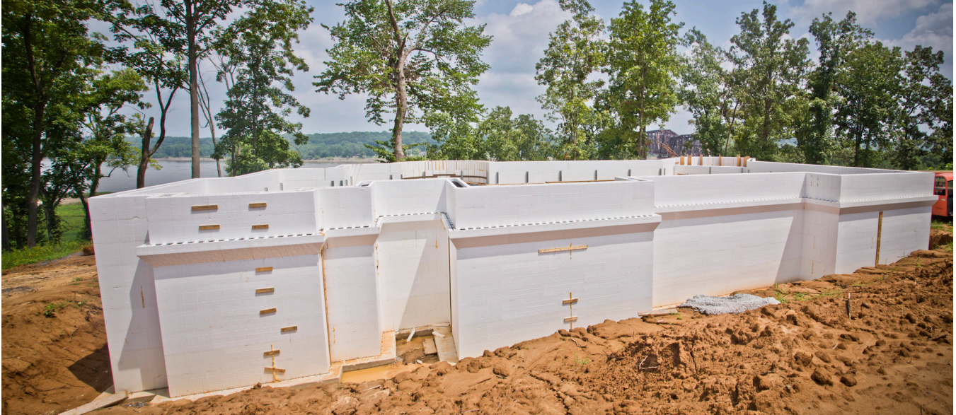
Figure 6.3.1 ICF walkout basement with brick ledge installed to support masonry veneer above grade.
