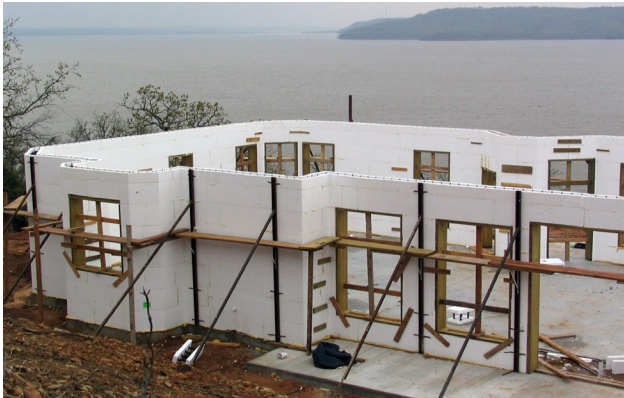
Figure 9.6.1 Minimal Outer Bracing
