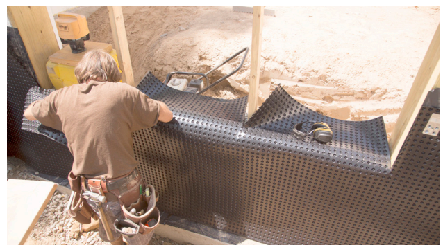
Figure 6.4.7 Extend waterproofing into window openings to ensure moisture cannot enter.
