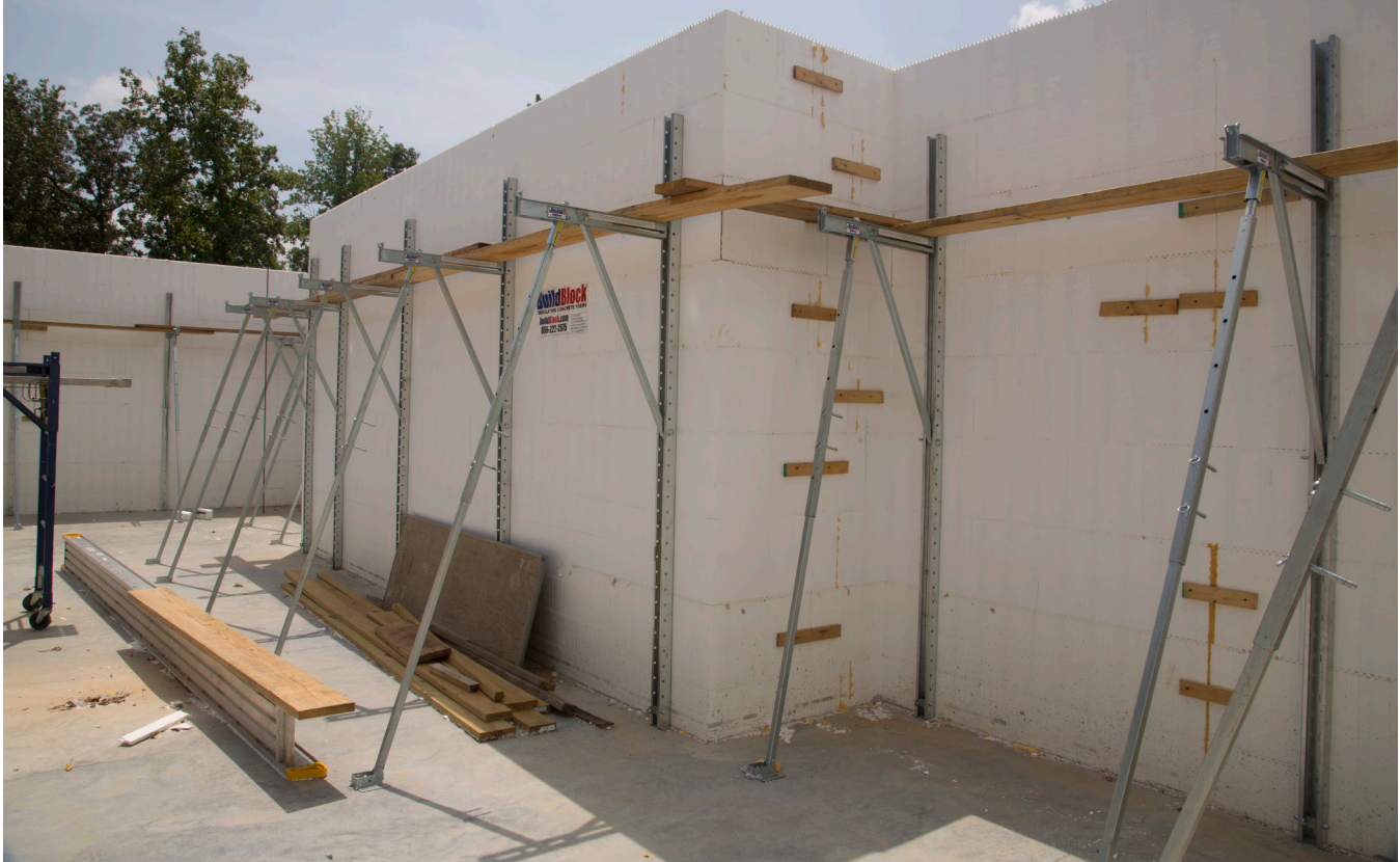
BuildBrace Build1 used in a residential project.
