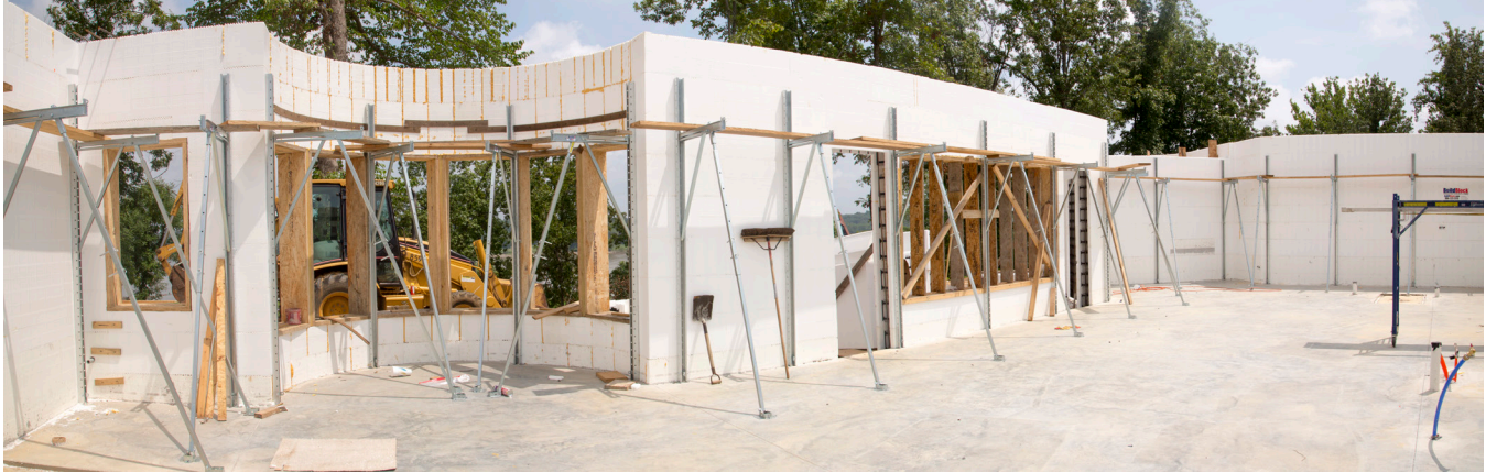
BuildBlock ICF Interior walls braced and ready for pouring.
