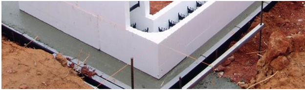
Figure 6.1.5 String lines used to ensure square and ICF form above corner forms locking corner in place until set.
