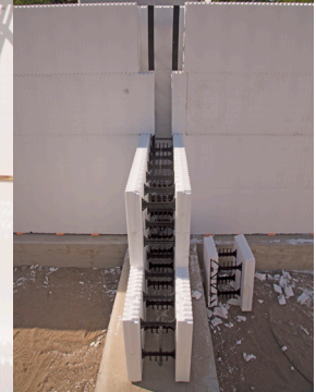
Figure 5.5.3 intersecting wall opening types.
