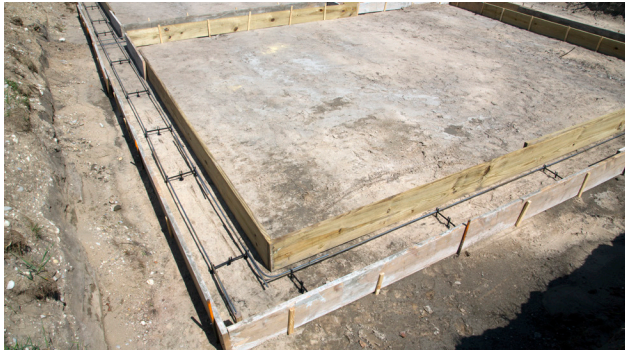
Figure 4.1.5 Formed footings with horizontal rebar placed in per local codes.
