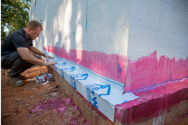
Figure 6.4.3 Installer placing a self-adhesive waterproofing membrane. Notice the 12" of membrane at the bottom of the wall sealing the footing to the wall.
