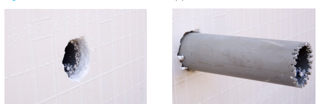
Figure 7.1.3 Cut small teeth on one end of the pipe sleeve and use to saw through the other side of the block to create a smooth opening.
