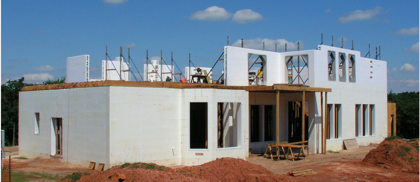
Figure 5.8.1 This partial second story has many openings, steps in height, bulkheads for wood frame attic, and is braced on the inside of the wall.
