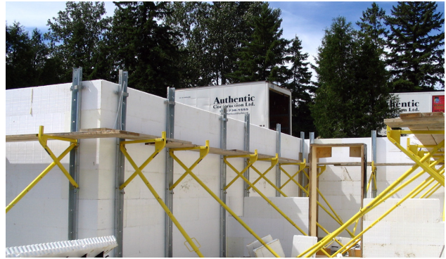
Figure 9.6.4 More Secure Inner Bracing w/ Walk Board
