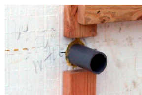
Figure 7.1.5 Add additional strapping if necessary, cut pipes flush after the pour for a seamless finish.
