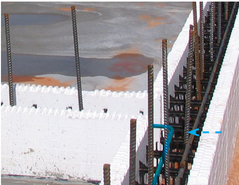
Figure 5.5.8 Intersecting wall opening types.
