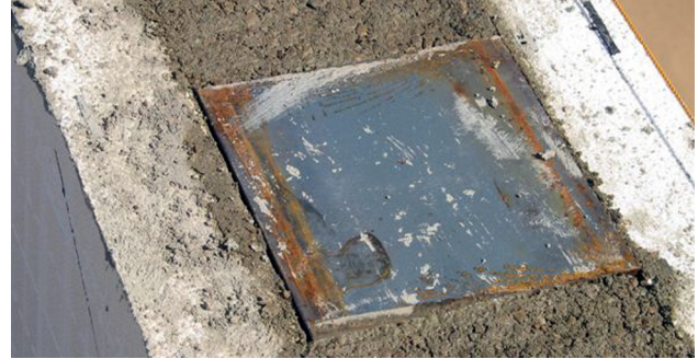
Figure 5.10.3 Steel bearing plate embedded into the top of an ICF wall. Ensure the correct height taking into account the interlock.
