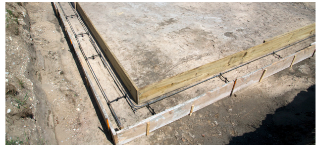
Figure 4.2.2 Formed and reinforced footings ready for pouring.
