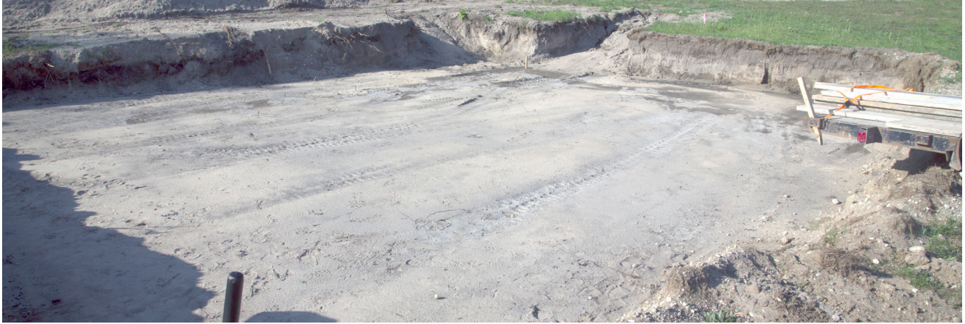
Figure 4.2.1 Typical site excavation staked for square
