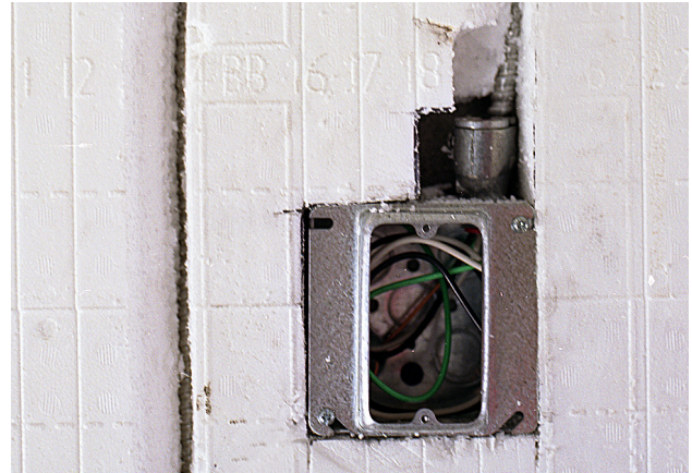
Figure 11.1.4 Electrical box with small wire chase cut in foam.
