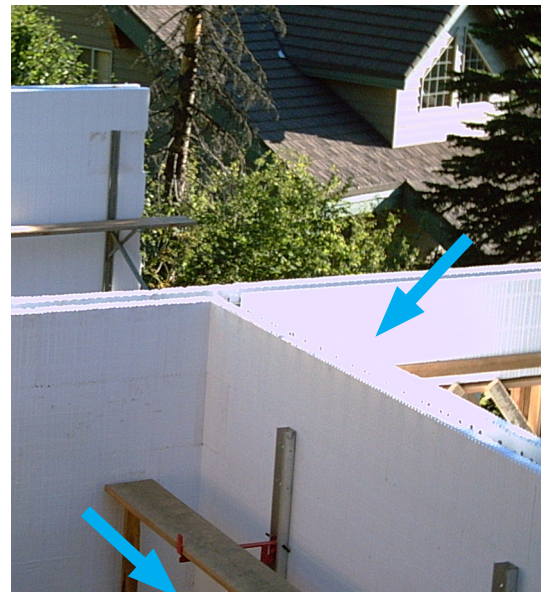
Figure 5.5.9 Intersecting wall opening types.
