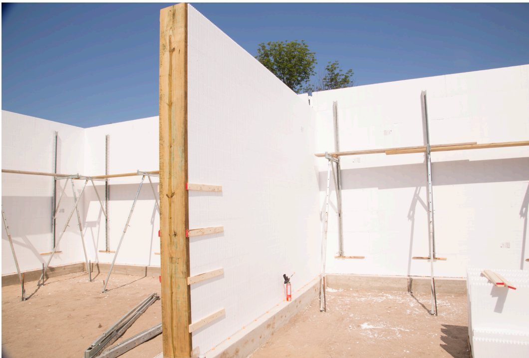
Figure 5.5.1 Intersecting Bulkhead wall with strapping.
