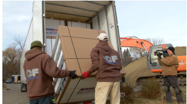
Figure 1.7.2 Unload BuildBlock forms flat to prevent damage to edges and corners.
