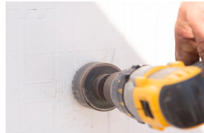
Figure 7.1.2 Drill hole the same diameter as the pipe sleeve to be used.
