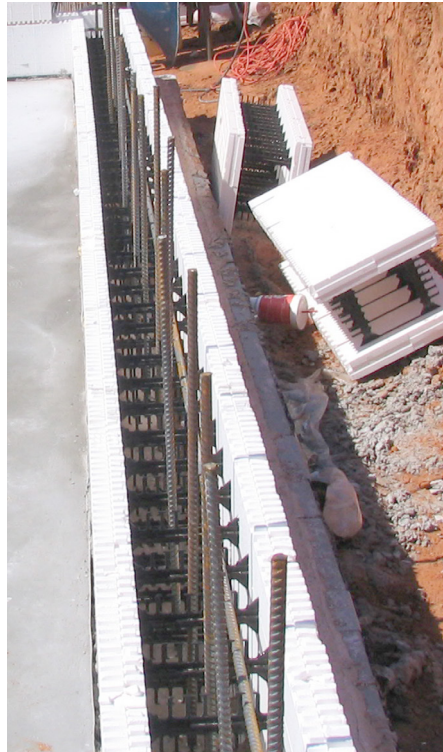
4.4.3 Wet set blocks placed with vertical & horizontal rebar .
