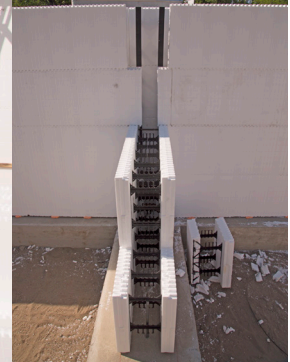
Figure 5.5.3 intersecting wall opening types.
