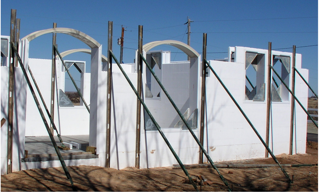
Figure 8.5.1 Arched windows and doors are easily integrated into BuildBlock ICF walls.
