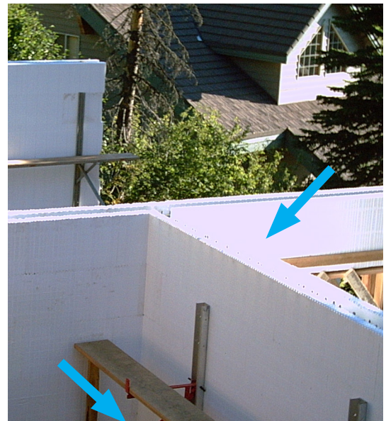
Figure 5.5.9 Intersecting wall opening types.
