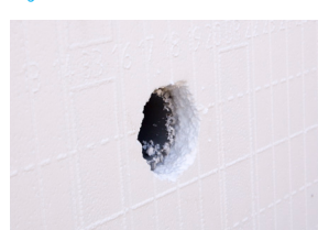
Figure 7.1.3 Cut small teeth on one end of the pipe sleeve and use to saw through the other side of the block to create a smooth opening.
