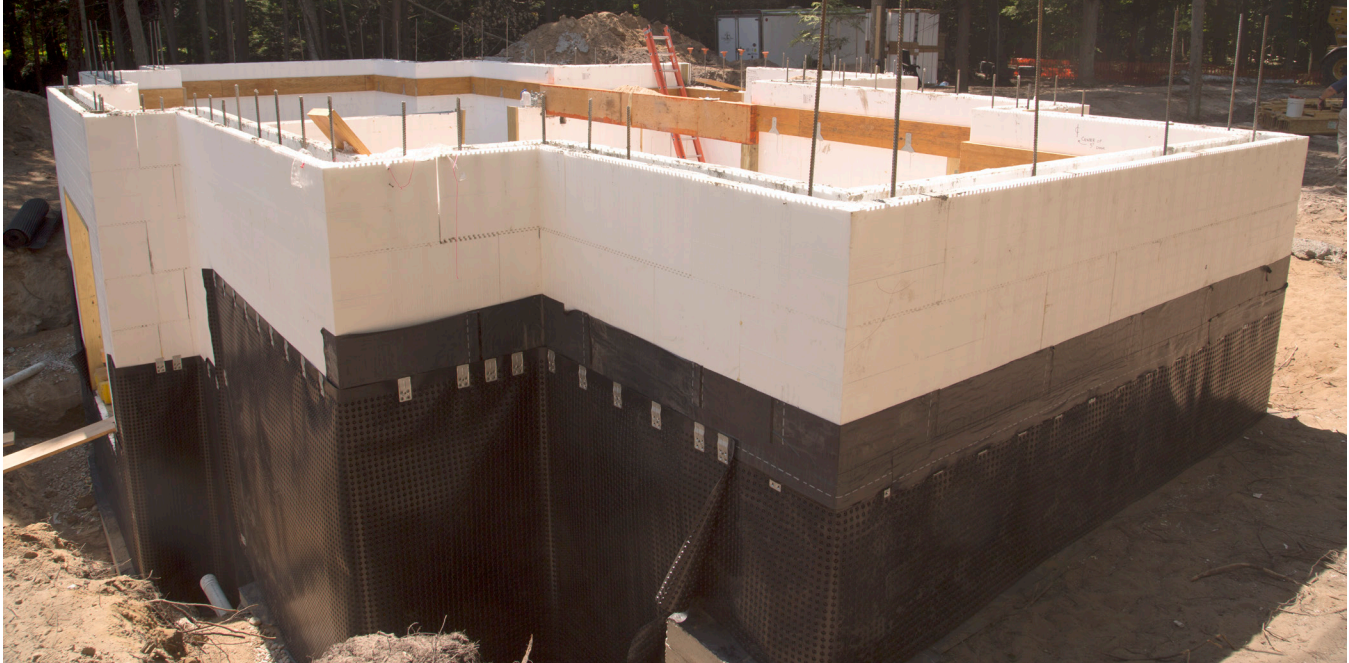
Figure 6.4.1 Below grade ICF walls with peel and stick membrane waterproofing applied and Air Gap barrier to prevent damage from backfill and provide hydrostatic pressure relief.
