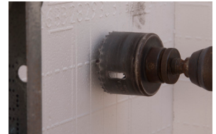
Figure 7.1.2 Drill hole the same diameter as the pipe sleeve to be used.
