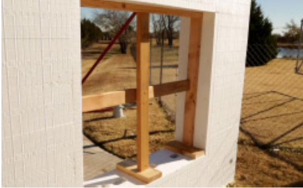
Figure 8.1.2 BuildBlock ICF bucking placed into the walls. Notice cross-bracing on corners to ensure it remains square.
