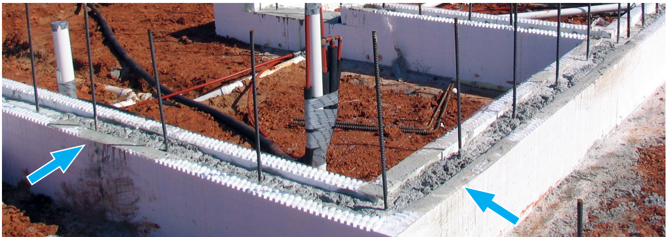
4.4.4 Wet set blocks placed with vertical & horizontal rebar for slab on grade applications in conjunction with stem wall construction. Leave concrete slightly rough 1-2" below tops of the blocks. Protect block interlocks to continue stacking additional courses.
