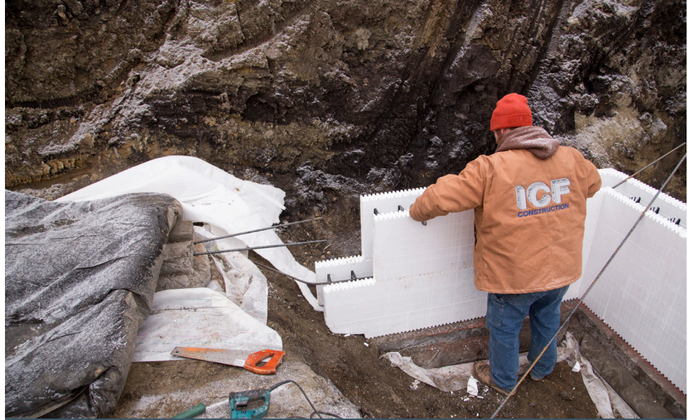
Figure 4.3.3 Building a Step Footing. Notice the horizontal rebar extending from the higher footing to tie the horizontal block to the footing.
