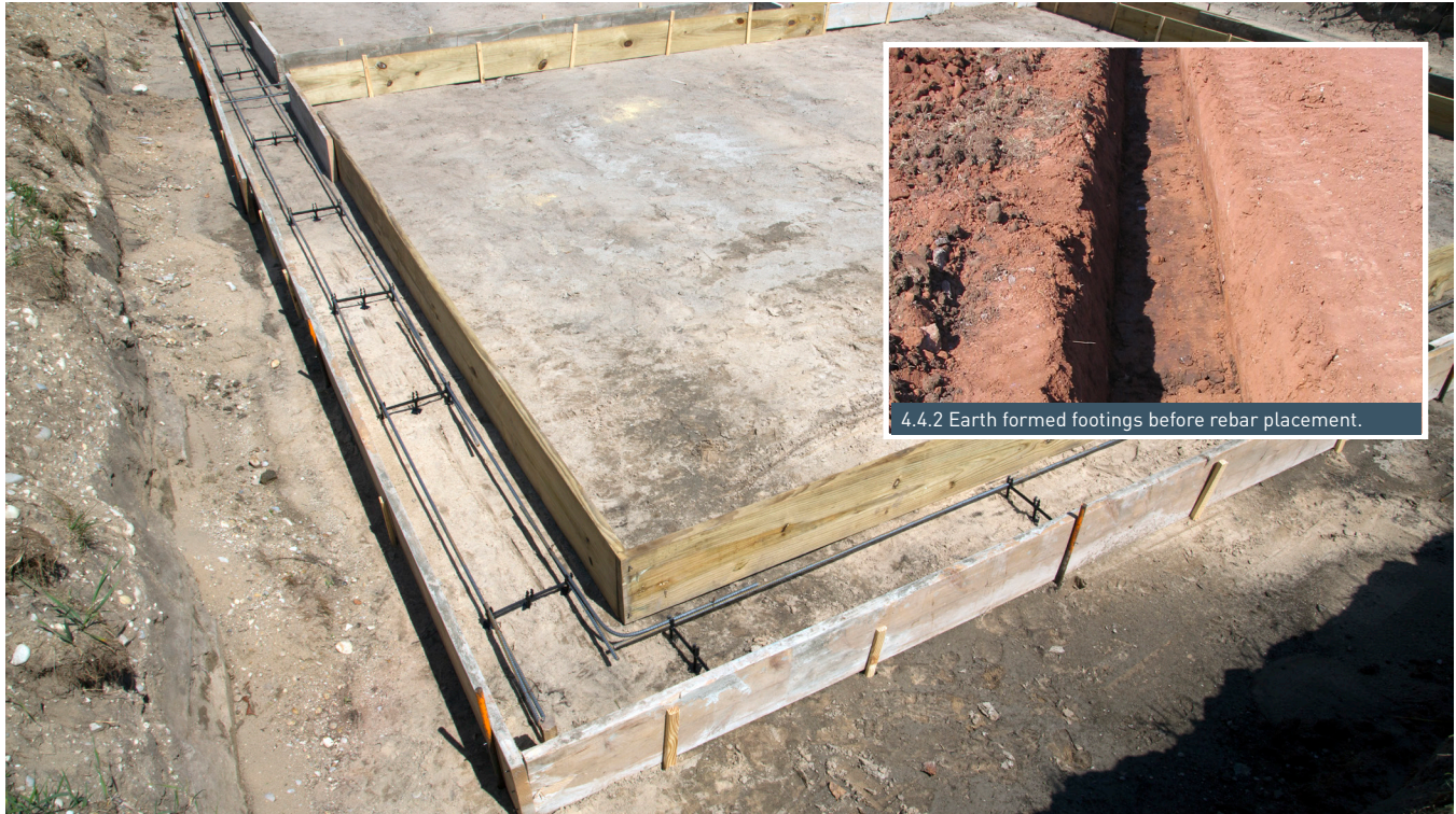
Figure 4.4.1 Footings formed with horizontal rebar in place.
