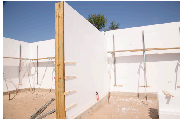
Figure 5.12.1 An end wall, properly bucked and strapped prior to installation of bracing & alignment system before concrete pour.
