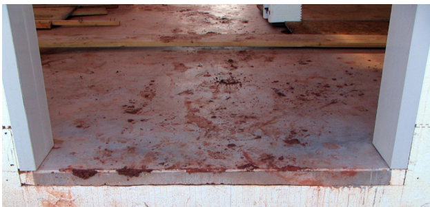
8.2.2 Note the concrete threshold poured to the outside wall edge. Bucking was properly braced during the pour to prevent any warping or cupping. Doors do not use bucking on the bottom of the door frame. Also notice the slab poured over the door threshold by cutting the block out 1-2" below the door height.
