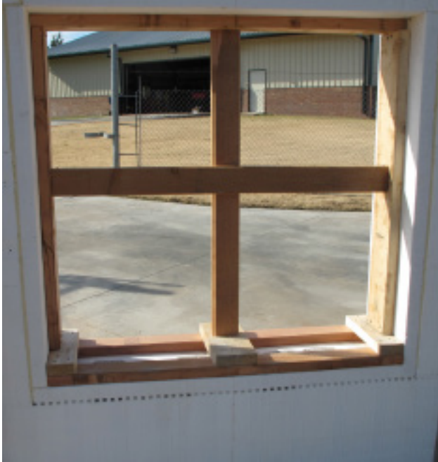
8.2.1 All bucks must be angle braced to keep them square and true.
