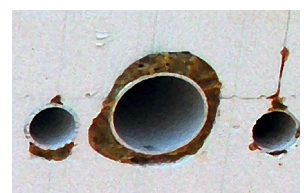
Figure 7.1.5 Add additional strapping if necessary, cut pipes flush after the pour for a seamless finish.
