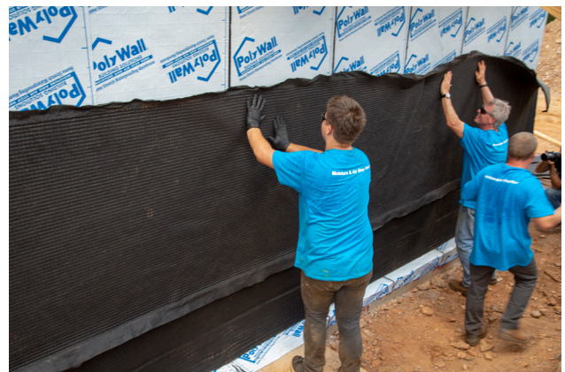
Figure 6.4.6 Arroyo Drain Board Waterproofing and air gap membrane is installed and brought at least 1-foot above backfill level. Comply with local codes.
