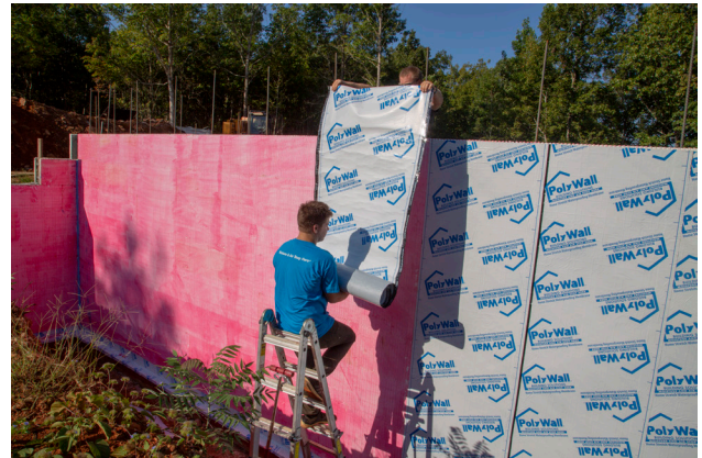
Figure 6.4.5 Poly-Wall Home Stretch Membrane is installed lapping seams at least 3" so water flows over the seam not against it.
