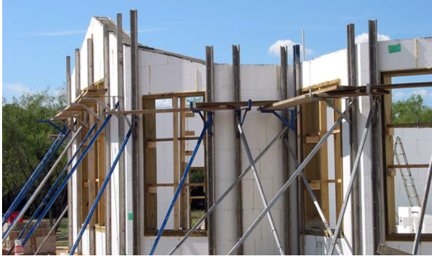
Figure 9.6.2 More Secure Outer Bracing
