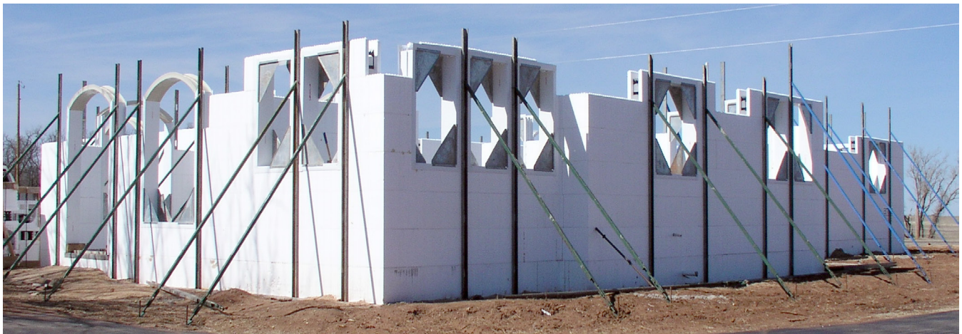
Figure 8.4.2 For larger openings than 3' wide, additional bracing and "bracing legs" (long 2x4 wood legs screwed to the vertical bucks and run to a base plate will help keep your openings straight and plumb during the pour.
