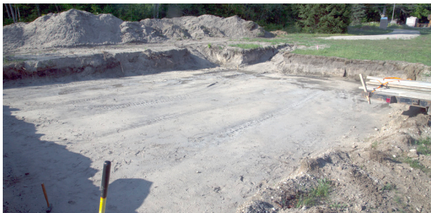
Figure 4.1.4 Excavated Footprint for footings.
