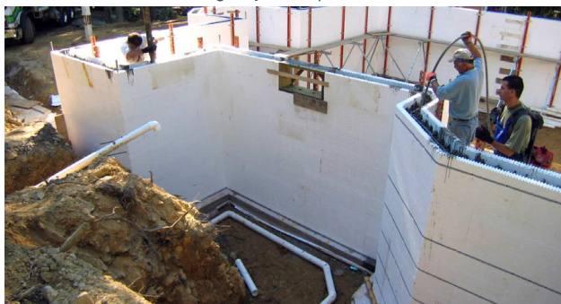
Figure 6.1.2 Standard french drain using slotted PVC pipe:
