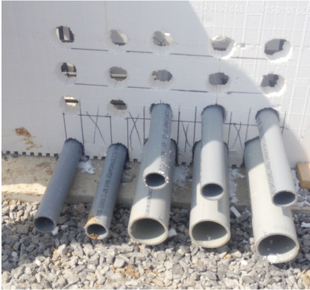
Figure 7.1.1 Complex service penetrations before additional strapping.
