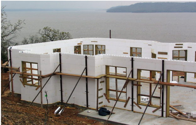
Figure 9.6.1 Minimal Outer Bracing
