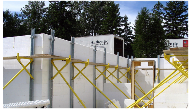
Figure 9.6.4 More Secure Inner Bracing w/ Walk Board
