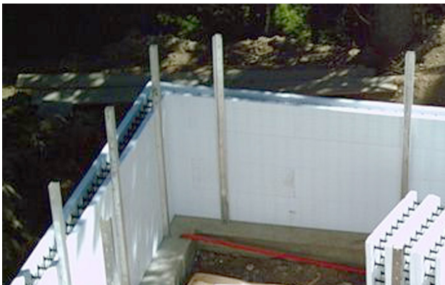
Figure 9.6.3 Minimal Inner Bracing
