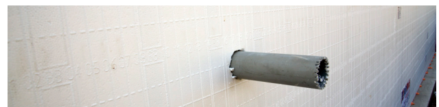
Figure 7.1.4 Secure any space around the pipe sleeve with foam adhesive before the pour.
