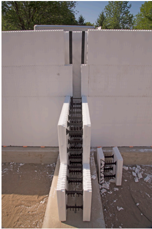
Figure 5.5.4 Intersecting wall opening types.
